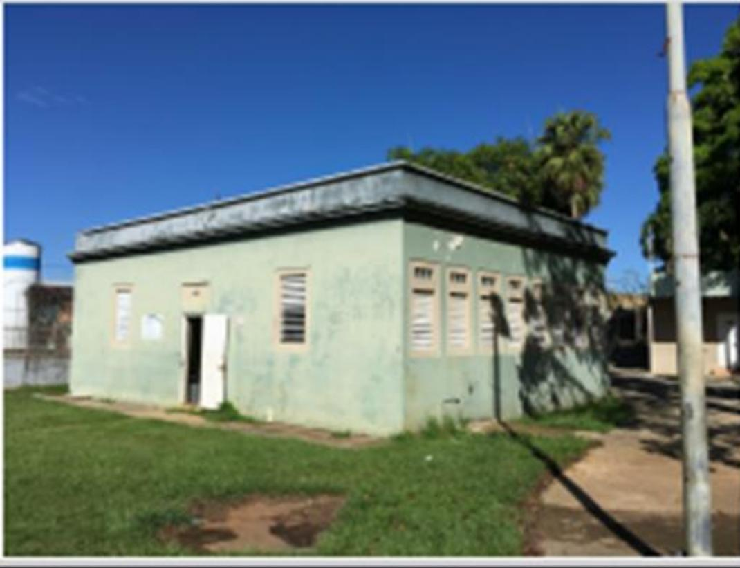
The Baños de Atletas building is a 1,300 SF, single-story bathroom and storage building that was constructed in 1940 (84 years old). The building is a cast-in-place reinforced concrete building with 3-FT parapets on three sides. The roof is sealed with an elastomeric coating. The interior includes reinforced CMU wall partitions. Interior finishes generally consist of plastered ceiling, plastered and painted walls and hydraulic floor tile.
