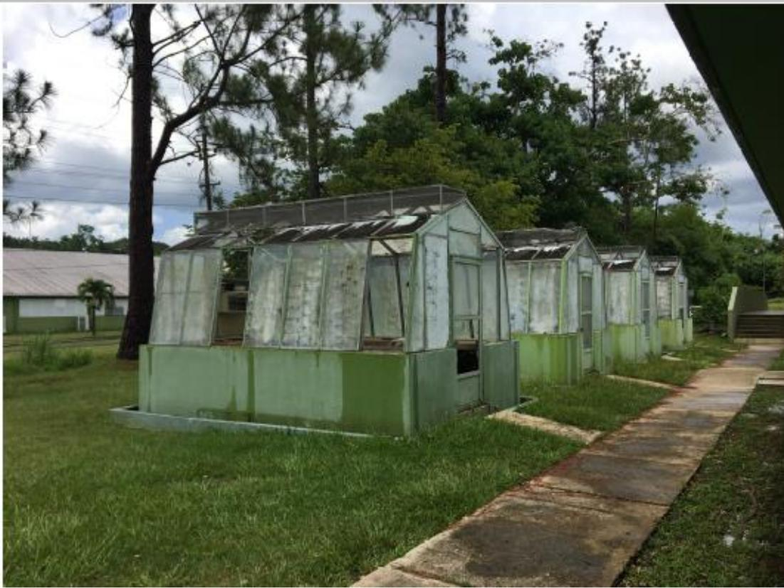
Greenhouses 1, 2, 3, and 4 have a 3-foot reinforced concrete wall supporting a metal frame structure. The roof (225 SF) is made up of glass panels. The interior finishes are made up of glass panels, bird screen, concrete walls and floor. The Greenhouses are located just north of the Entomology Lab.
